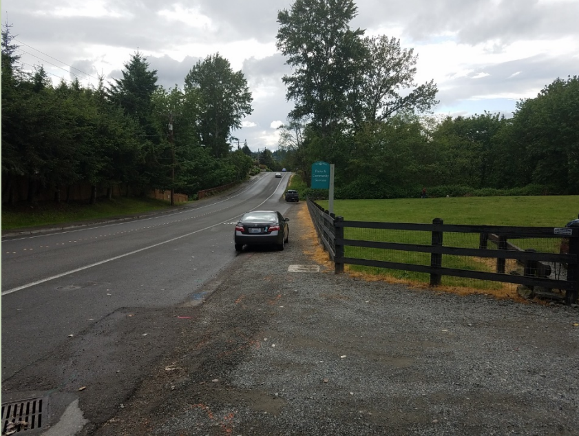
SE 60 th St. ROW looking West
