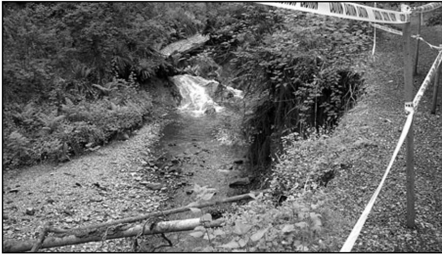
Stream boulders, logs and root wads have been installed along Coal Creek to prevent erosion and enhance fish habitat.
