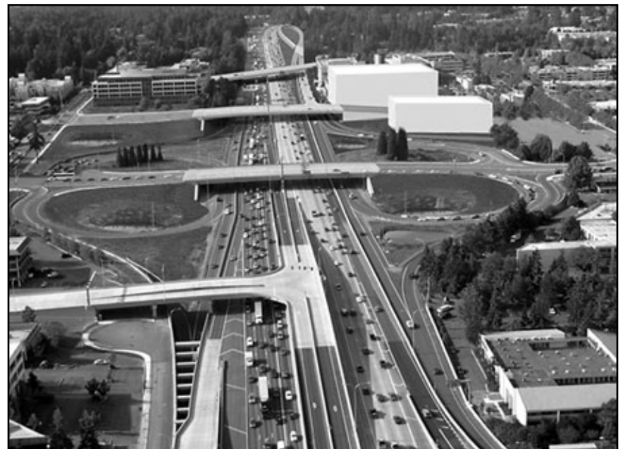
This visualization shows the addition of both the Northeast 10th Street Bridge and the braided on- and off-ramps.
