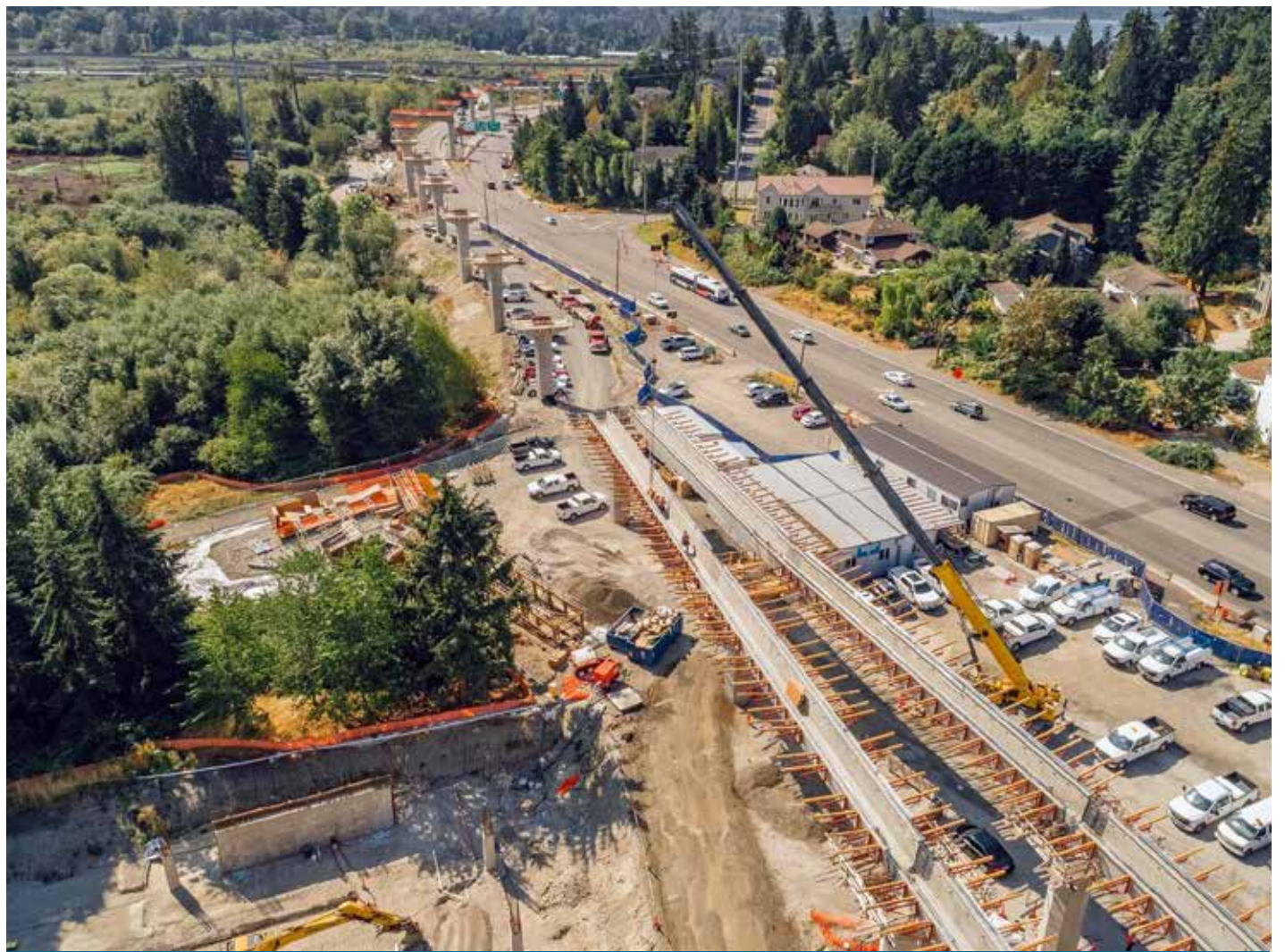
Aerial view of East Link construction in South Bellevue.
