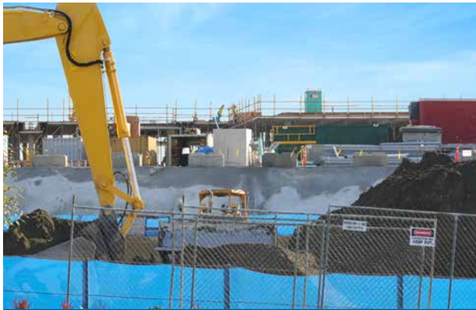
Construction in the Spring District.
