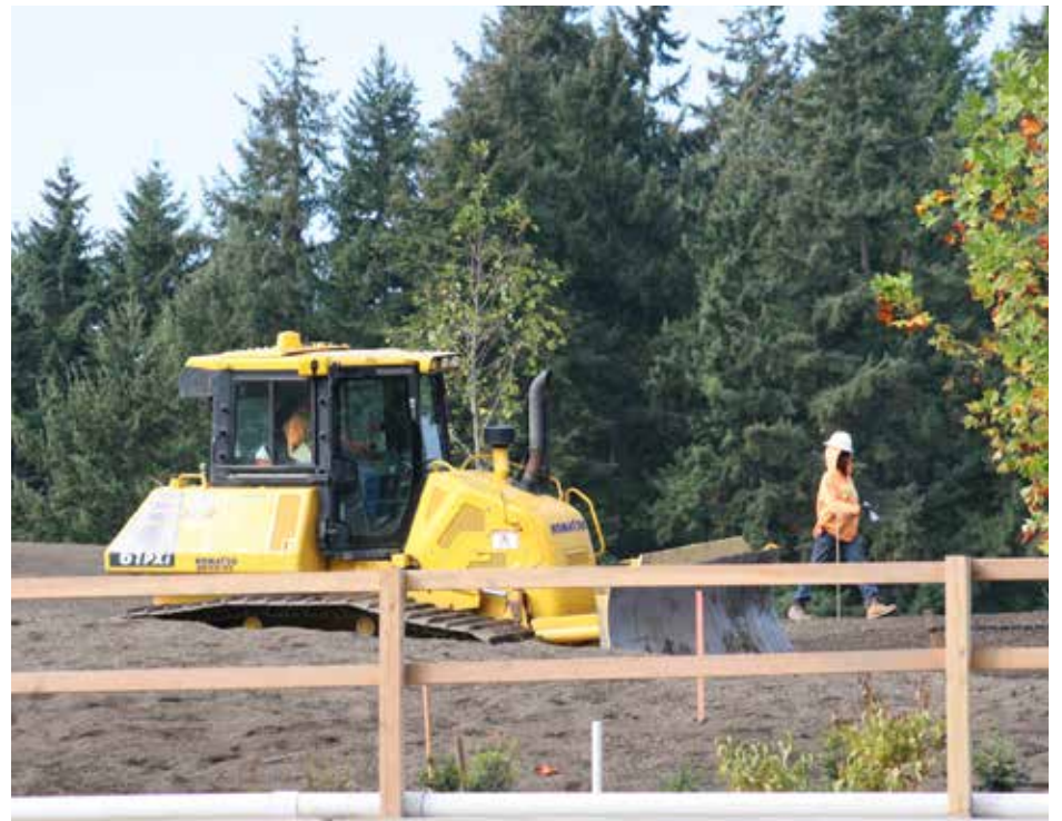
Landscaping for Surrey Downs Park progresses
