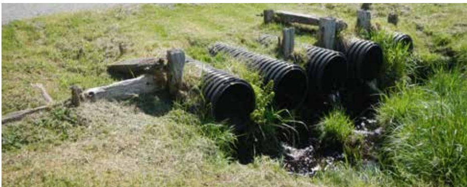
A pedestrian bridge will replace these culverts.
