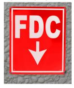
The location of the FDC's may not always be visible from the street or nearest point of fire apparatus access. In those instances, the location of the connection must be clearly identified with approved signage. The letters "FDC" must
