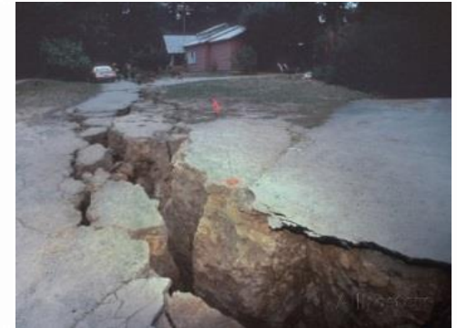
Loma Prieta, CA 1989
