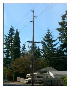
Utility pole carrying transmission wires (top section), distribution wires (middle section), and telecom wires (lower section)
