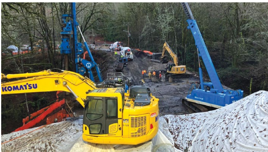
Early days of construction for a bridge on Lakemont Boulevard.
