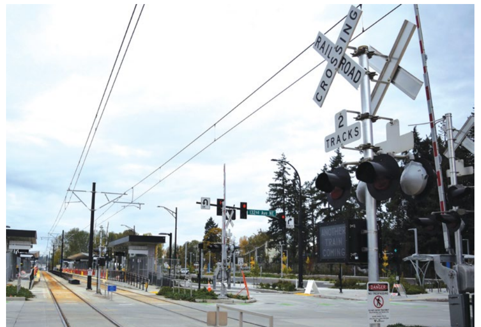
People should be extra careful at light rail crossings like this one in BelRed.
