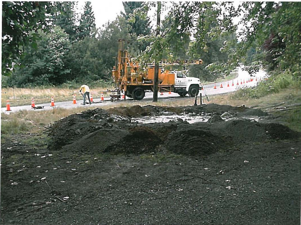
Photograph 10 - Drill cutting stockpile and concrete waste clean out area.
