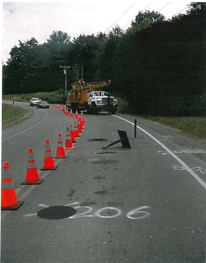
Photograph 8 - Patched drill hole and steel plate hole cover prior to placement.
