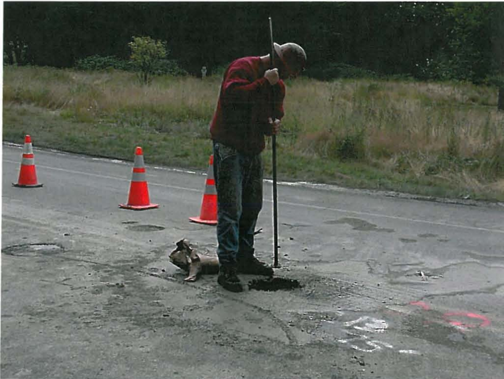
Photograph 7 - Patching drill holes.
