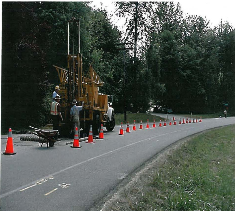
Photograph 2 - Looking south. Drilling in northbound lane.
