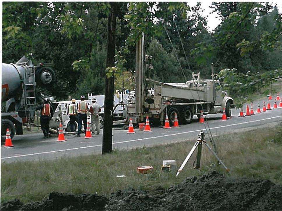
Photograph 4 - Grout placement. Looking northwest. OSM optical survey monitoring setup in foreground.
