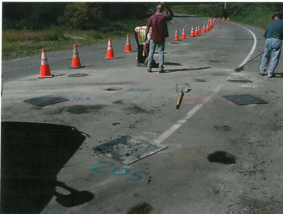
Photograph 6 - Daily clean up. Hole cover plates in place.
