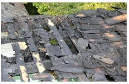
**August 9, 2018** – Spontaneous combustion of an oil-soaked rag used to stain a deck the previous day caused extensive damage to the roof of the attached dwelling.
