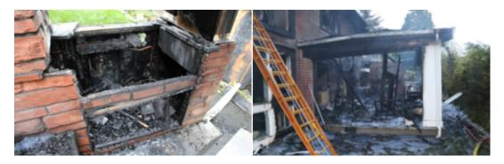
**May 24, 2018** – A barbeque left on overnight and installed closer to combustible materials than required by the manufacturer caused significant damage to the outdoor covered area and the interior of the residence.
