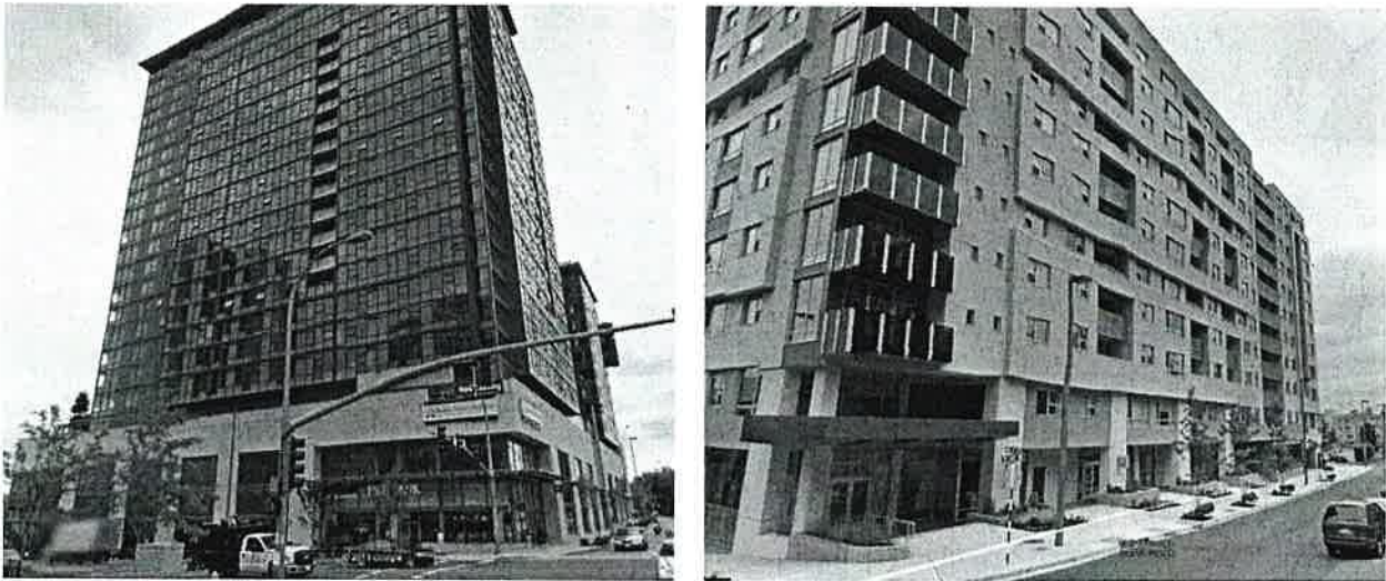
FIGURE 20. Both of these wide buildings could have used design elements to more effectively break up the massing and add interest. Avalon Towers (left) could have used features both to break up its Bellevue Way base (lower floors) and its tower. The M112 building incorporated color changes and other small scale articulation features, but the façade in this view still comes across as very flat.
