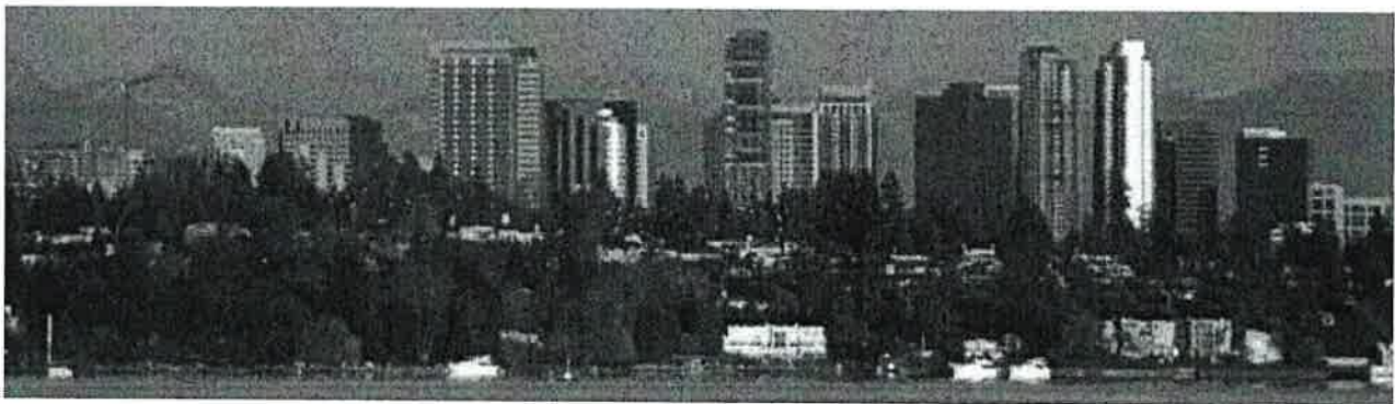
FIGURE 15. Downtown's skyline, when viewed from a distance, lacks much visual interest in terms of rooftop forms.
