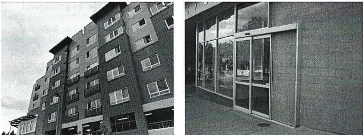
FIGURE 14. The use of concrete block (both images) and metal siding (left image, upper floors) also warrants discussion.
