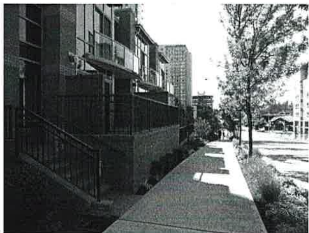
FIGURE 6. Washington Square townhouses provide landscaping and "eyes on the street".
