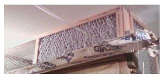
A disconnected dryer vent led to lint accumulations in a storage room of a multi-family building. In the same building, smoke detectors were missing in the bedrooms and a number of smoke detectors in other locations lacked batteries.
